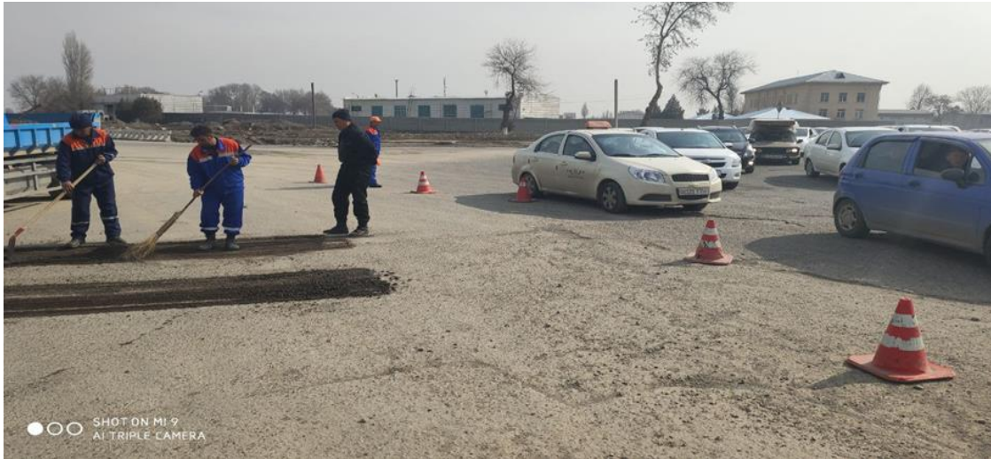
Figure-6. Condition of road markings and guardrails on the road section under repair.
