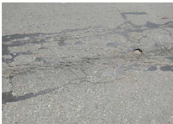
Picture 5. The process of turning cracks into grooves
