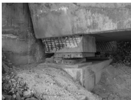
Damage to the abutment: offset of the hinge of the bearing part and damage to the abutment stone
